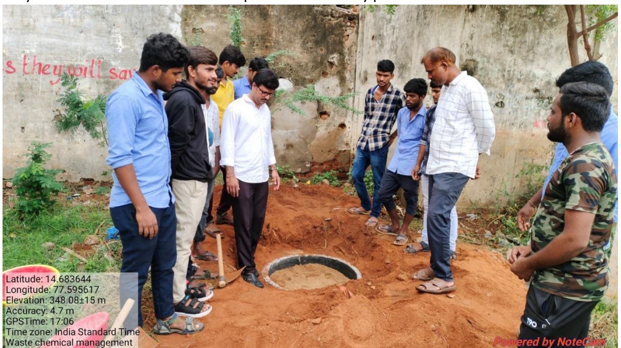
Pit made to dispose dissolved chemical substances
